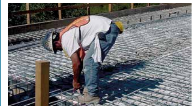
Bild 10-15. Hot galvanized reinforcement in bridge.
