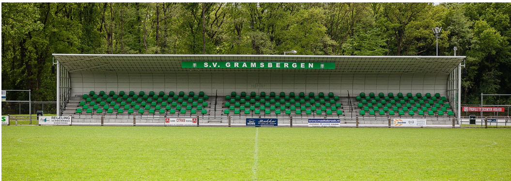
Left The reconstructed stand at SV Gramsbergen ready for another life cycle for its galvanized steel that could reach 100 years in total
